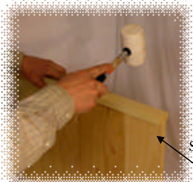
STEP 1: Drive tongue and groove panels together with mallet.
