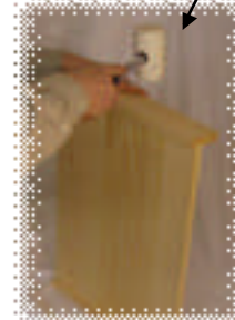
STEP 2: Drive end rail onto tongue and groove panel.
