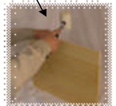
STEP 1: Drive tongue and groove panel together with mallet.
