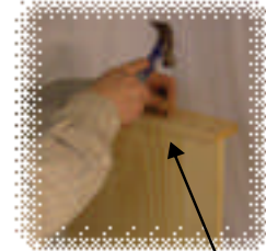
STEP 3: Nail end to tongue and groove panel with 6d sinkers.— 2 nails per panel
