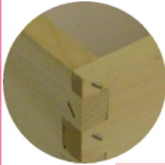
Close-up of Finger Joint
